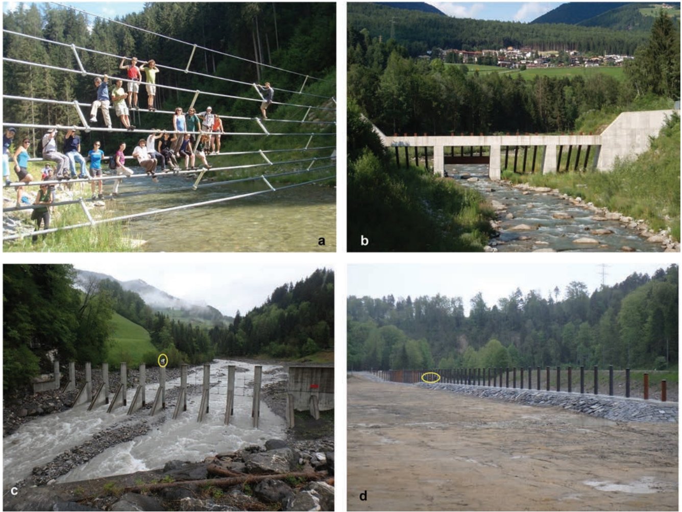
Figure 6. Examples of structures used to limit downstream mobility of wood. (a and b) Rienz River, Italy; (c) Chiene River, Switzerland (the chair is outlined in yellow for scale); (d) Sihl River, Switzerland (people are outlined in yellow for scale). The structure on the Sihl River is unique in size and design. It is installed parallel to the flow in the outer bend of a meander to retain wood (which might otherwise reach the City of Zurich) but to allow sediment to be transported.
