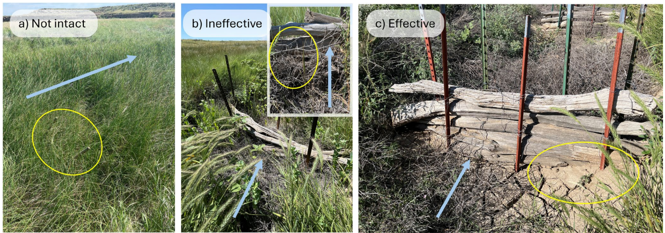
FIGURE 4 | Categorization of log-based erosion control structure outcomes as (a) not intact, (b) intact but ineffective, not resulting in detectable geomorphic change, and (c) intact and effective, resulting in detectable geomorphic change. Blue arrows indicate flow direction. [Color figure can be viewed at wileyonlinelibrary.com ]
