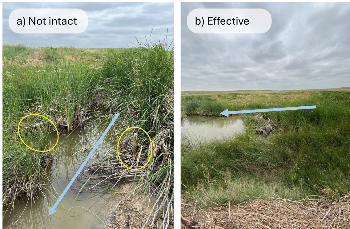
FIGURE 5 | Categorization of beaver dam analog (BDA) outcomes as (a) not intact and (b) intact and effective, resulting in detectable geomorphic change. Blue arrows indicate flow direction. [Color figure can be viewed at wileyonlinelibrary.com ]
