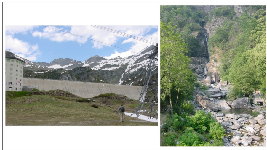
Fig. 11. Example of hydroelectric development in headwaters; here, the Maggia Valley in Switzerland, showing the dam at a glacial cirque (left) and the de-watered channel downstream (right).
