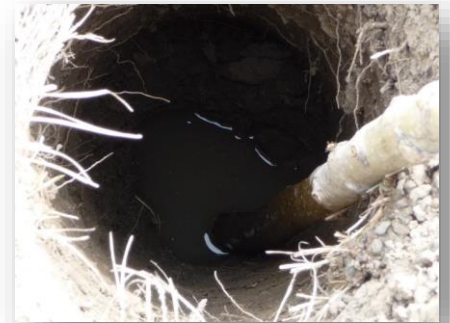
Image 4. Cottonwood pole in 8' deep pre-augered hole prior to slurry fill.
