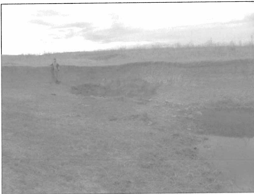
Figure 2. Upstream view of a collapse feature along South Pawnee Creek on the Pawnee National Grassland. Photograph taken in October, when the channel is dry but for refuge pools (upstream edge of pool in lower right corner of photo). Notice the unchannelized swale upstream.
